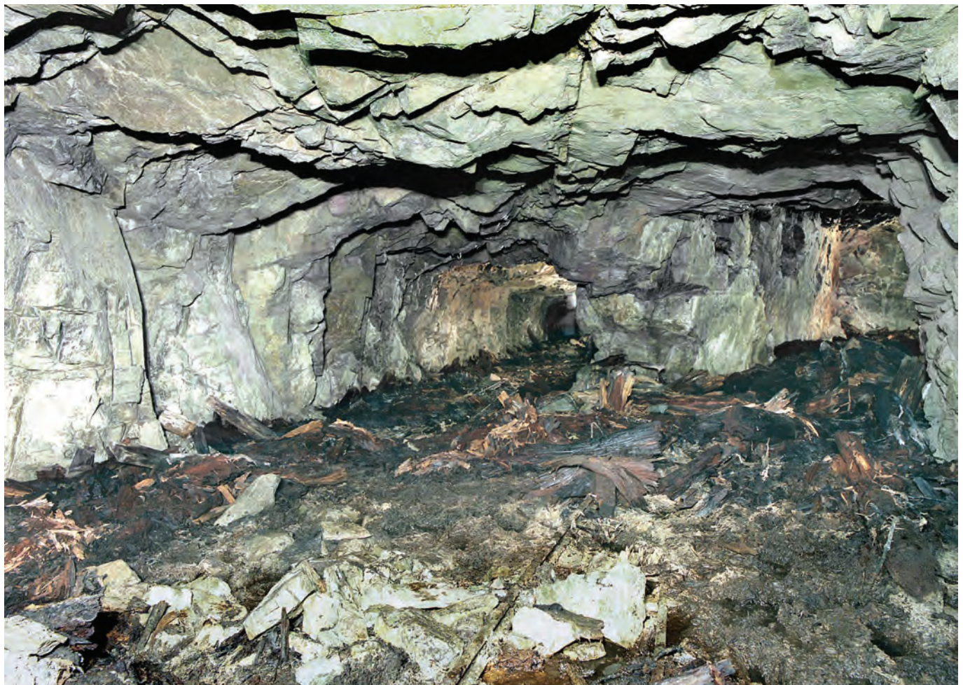
Junction of two tunnels in Water Lane Tunnel East (Ho 5) in Alderney. This former fuel storage tunnel and electricity generating station is difficult to negotiate as the floor is up to 18” deep in sludge.
